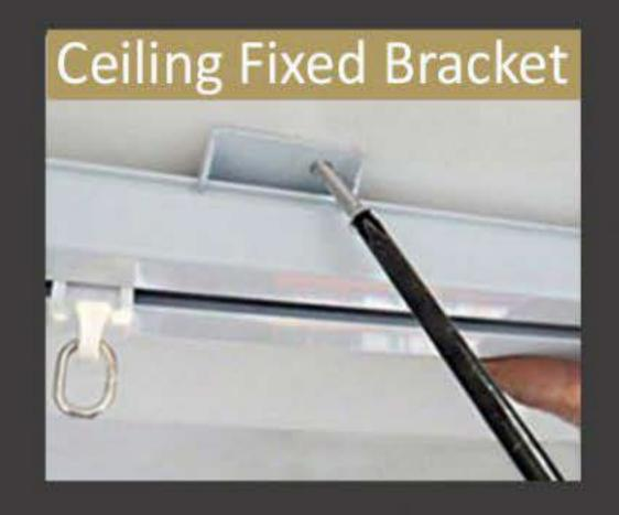
Select Ceiling Fixed Bracket if you are installing your curtain track to the ceiling
